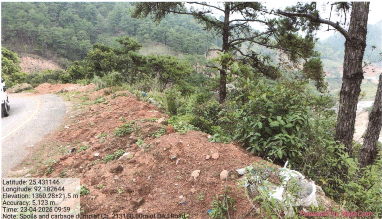
At Ch. 213180.00m of DAJ Road (NH-40E)
