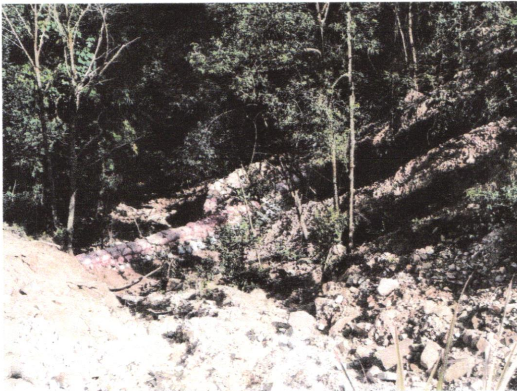
At Chainage: 3100.00m
