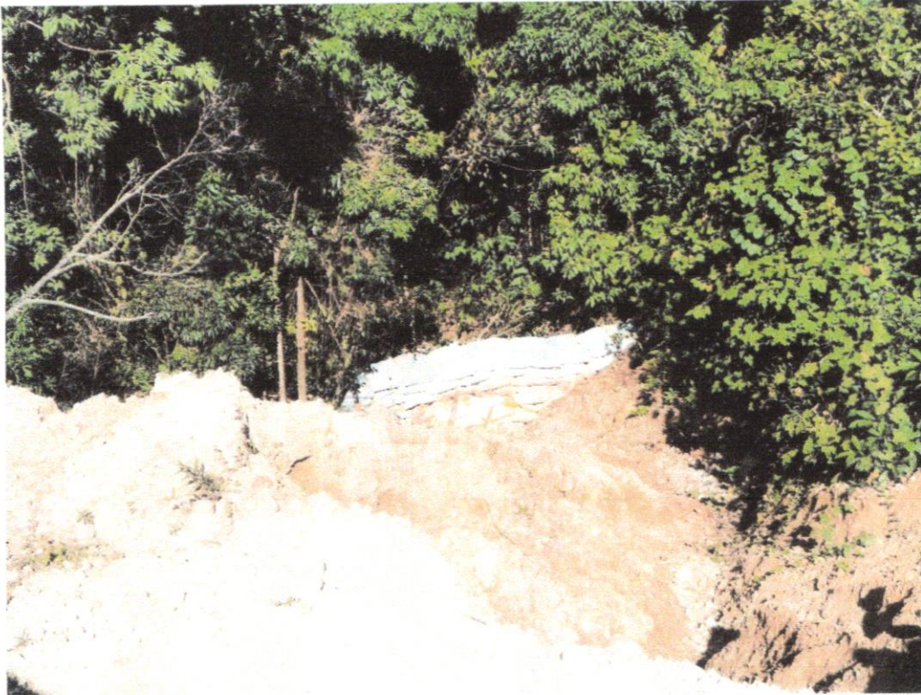
At Chainage: 4140.00m
