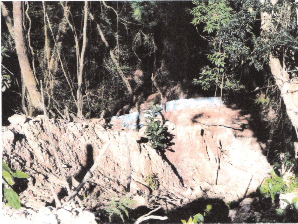
At Chainage: 2980.00m
