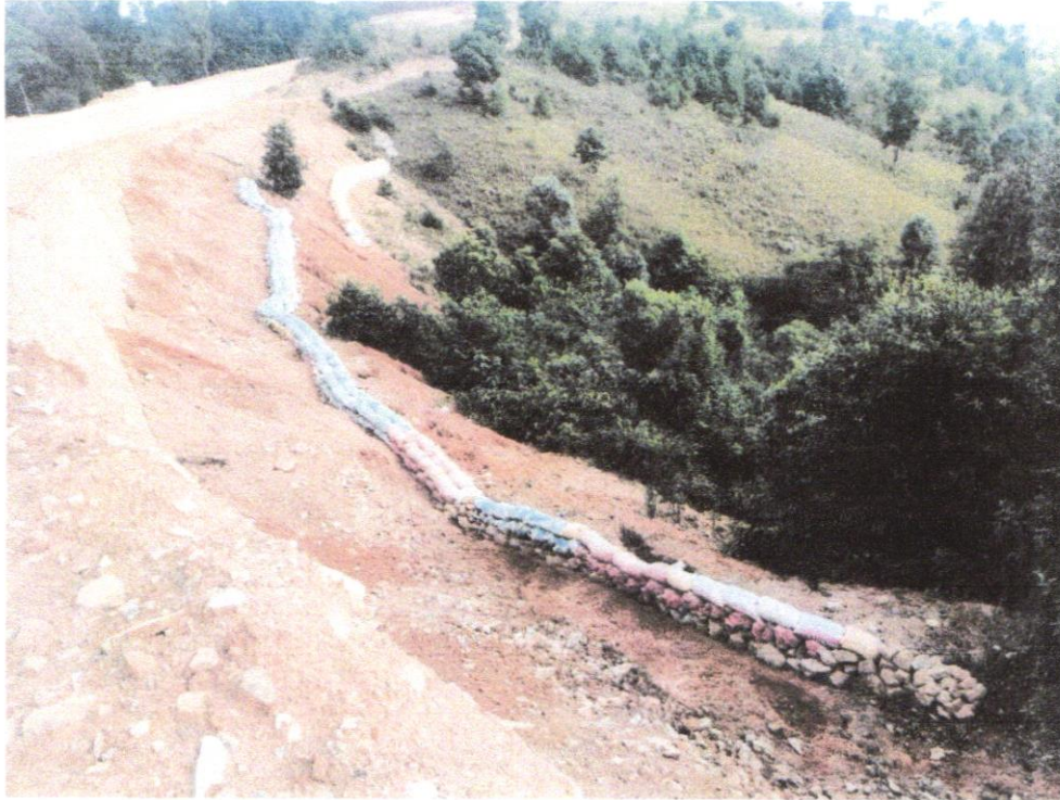
At Chainage: 4520.00m
