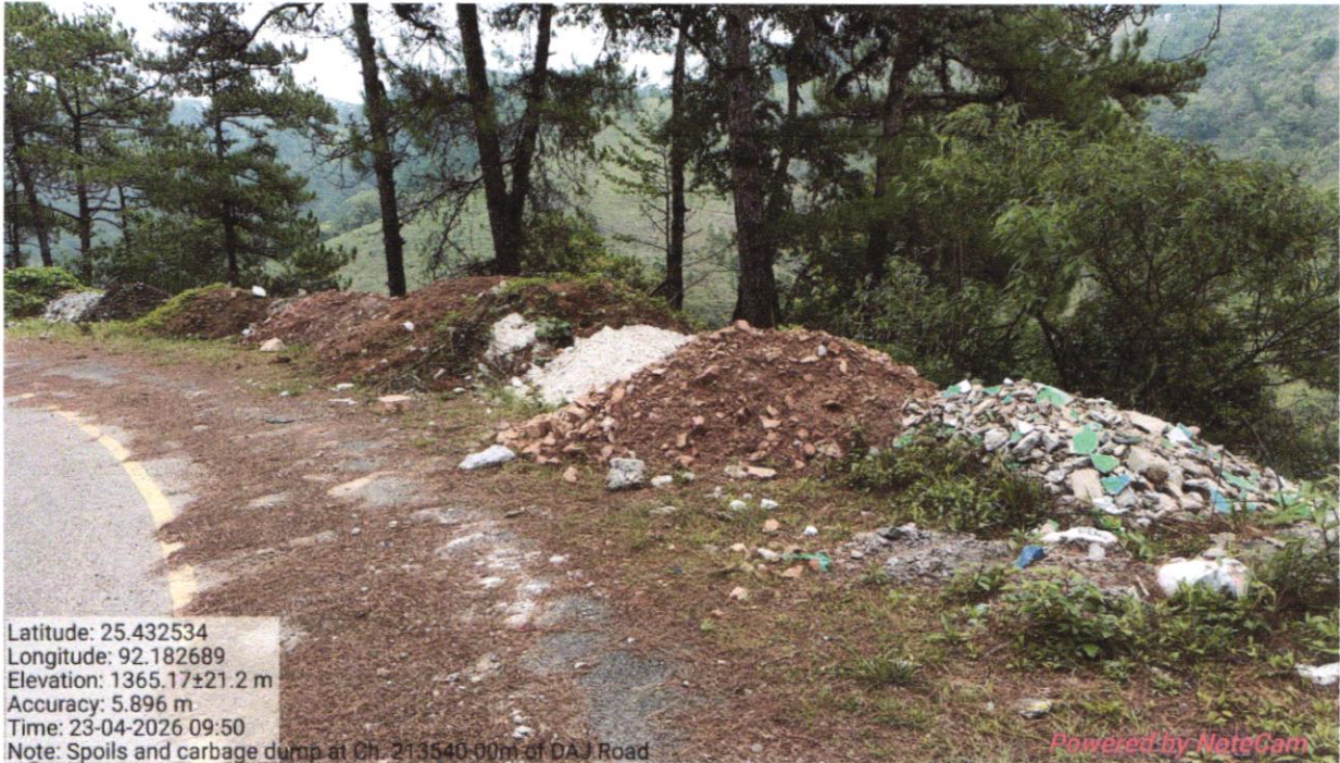
At Ch. 213540.00m of DAJ Road (NH-40E)
