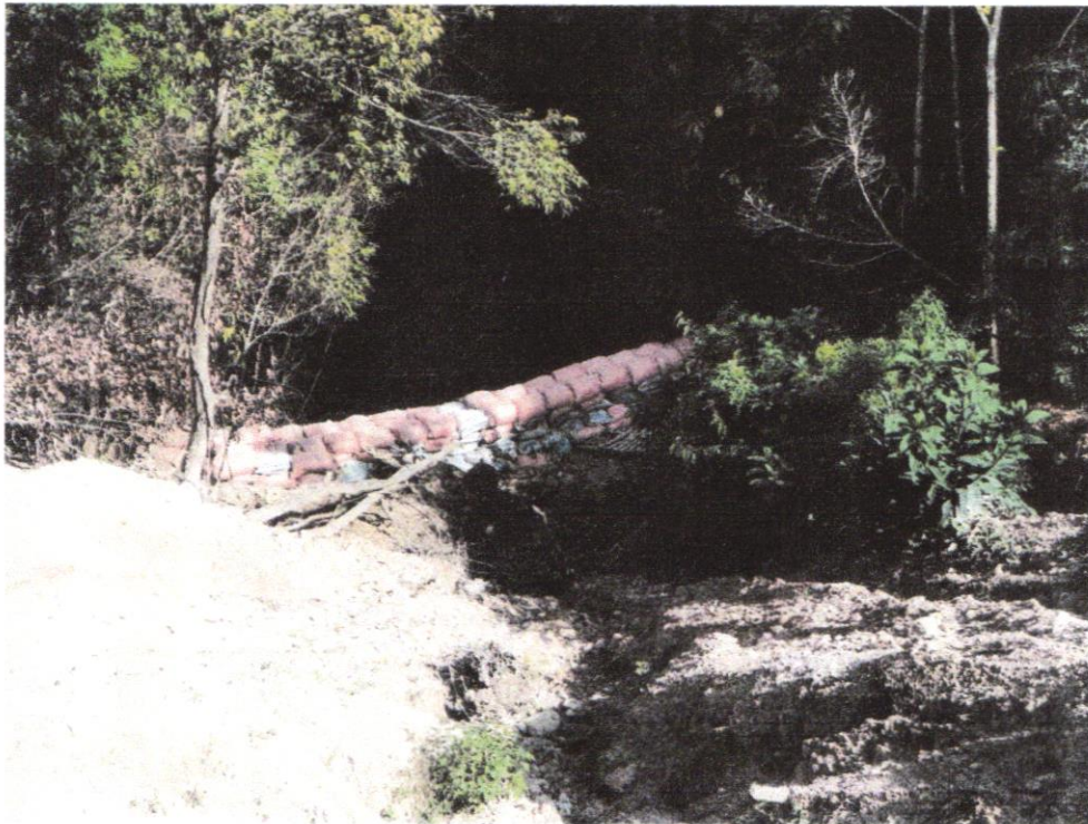
At Chainage: 4210.00m
