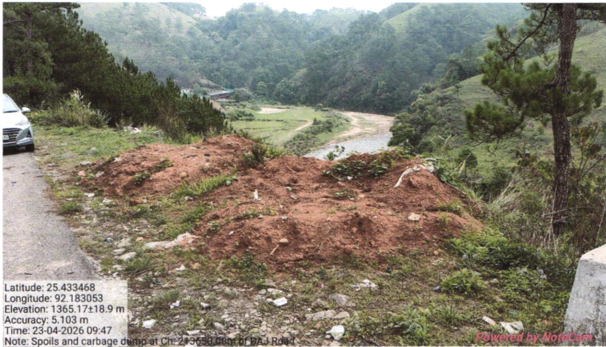
At Ch. 213650.00m of DAJ Road (NH-40E)
