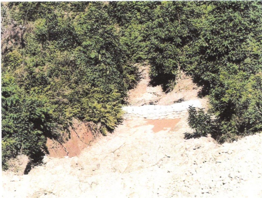
At Chainage: 3100.00m
