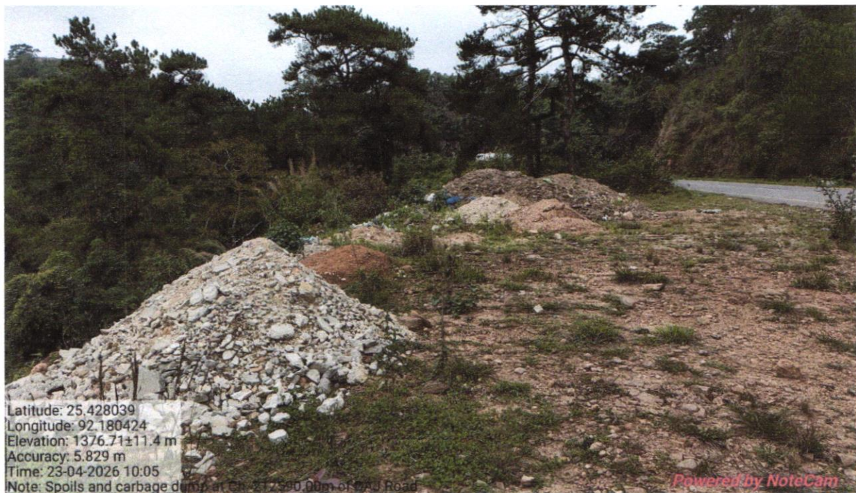
At Ch. 212590.00m of DAJ Road (NH-40E)
